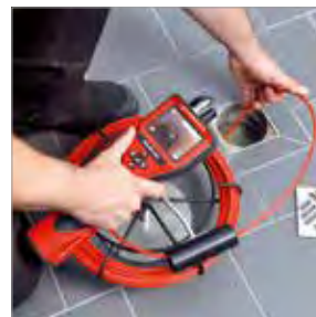
Inspection of floor drains
