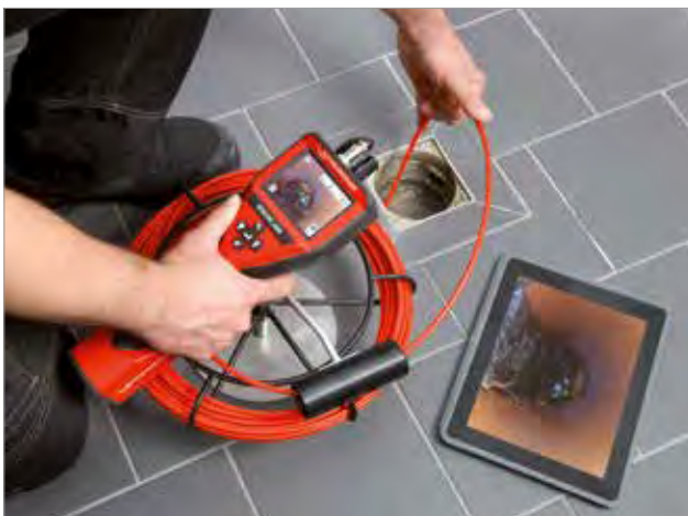
Inspection of basin drains
