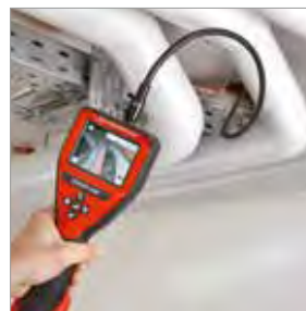
Inspection of hollow spaces
